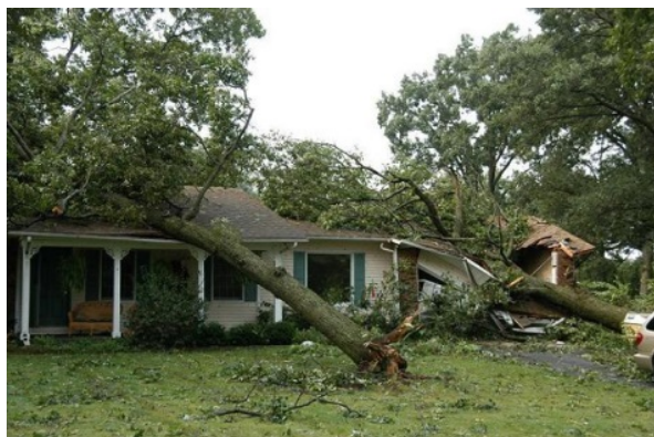
Figure 3-18 Home Damaged During Windstorm
